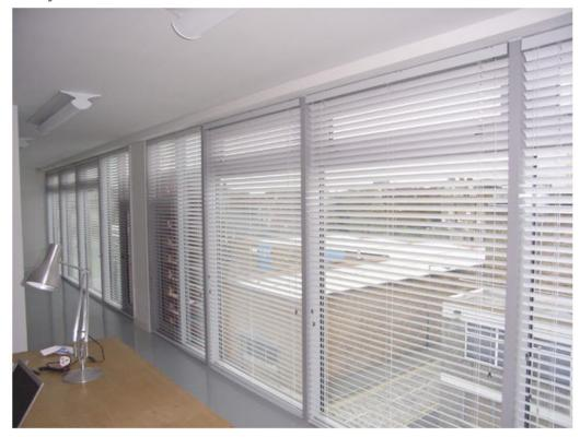
The Slimstyle blind has been engineered and developed to provide the widest possible range of control and installation options. Slimstyle features an exceptionally robust and compact headrail and can be used with either 16mm or 25mm slat.
