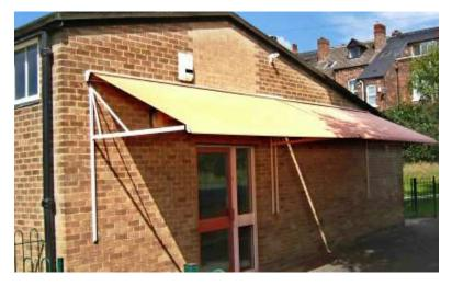
Sliding arm awnings operate the same way as a drop arm except that the pivot point moves up as the blind drops. There are three versions in our range with projections of 1650mm and 1950mm. This allows a longer projection and better head clearance under the arms. A spring provides resistance to wind buffeting.
