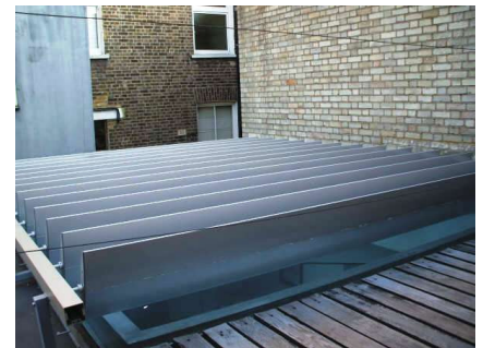
As external rooflight shading system.
