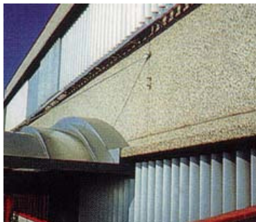
As an externally mounted vertical shading system.
